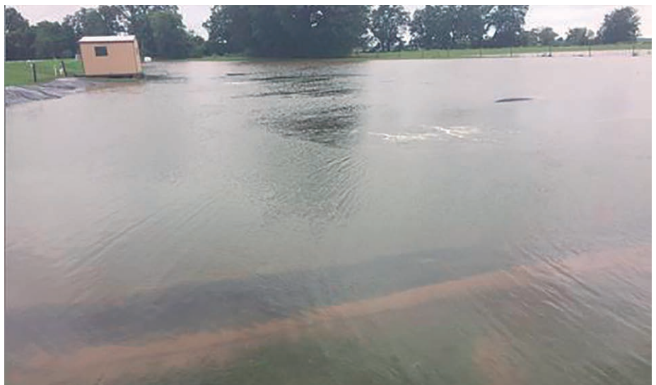
Low levees can be overtopped from flooding in the surrounding watershed. In this instance the pond liner and levee surface are visible, as is air bubbling up from diffusers supplied by an emergency blower located on the platform.
