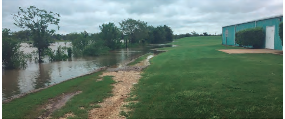
An example of placing hatchery buildings on constructed earthen raised platforms well above historic flood levels. The leveed pond complex is visible in the distance, behind the building.
