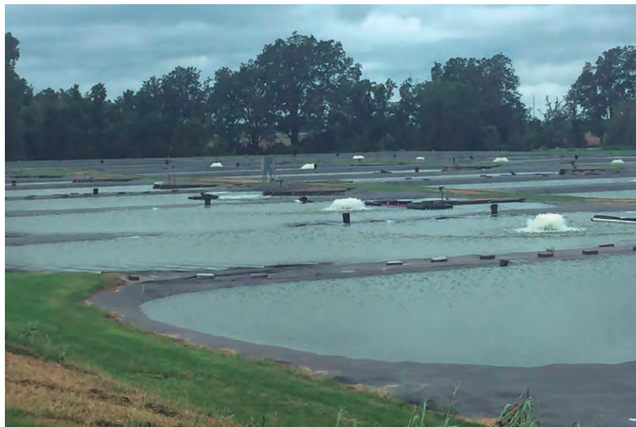
Pond topping and mixing, due to improperly sized drains incapable of handling heavy rainfall associated with hurricane events.
