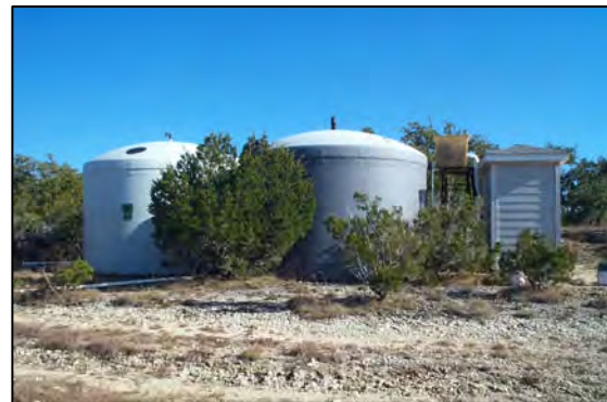
Figure 2-5. Two 10,000-gallon fiberglass tanks
