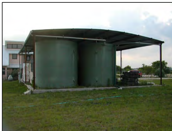
Two 10,000-gallon cisterns collect rainwater at the Pomerening/Dunford residence in Bexar County.
