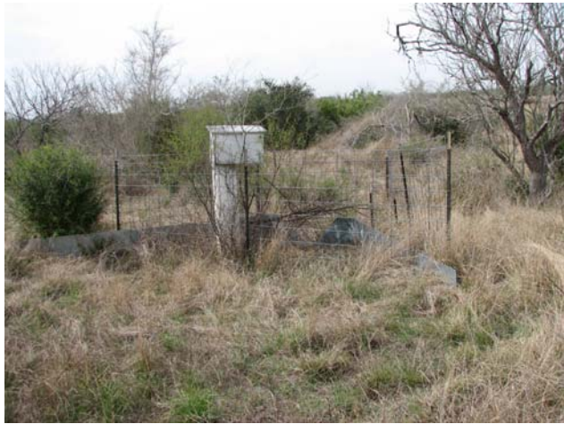
Figure 5. Site WWR-3 on February 26, 2007 prior to initiation of work to refurbish sites.
