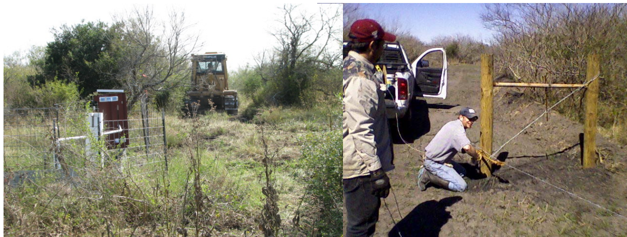
Figure 9. Brush clearing and berm reconstruction at WWR-3 on November 7, 2007 (left frame). Fence construction at WWR-1 on February 13, 2008 (right frame).
