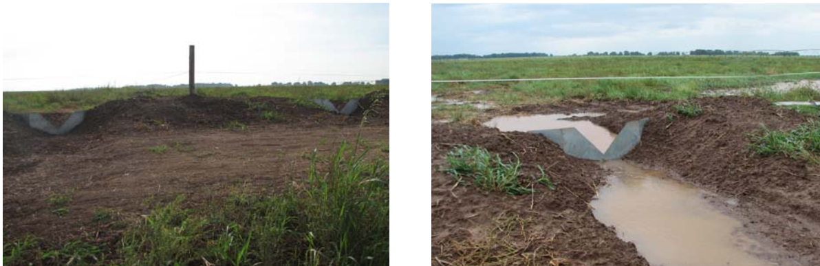
Figure 16. Electric fence and weirs installed on September 15, 2008 (left pane). Seepage under weir following a 4.25" rain from Hurricane Ike (right pane).
