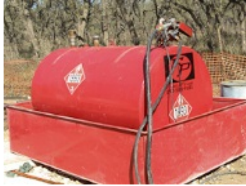
Figure 2: Metal or plastic containment pans are an inexpensive way to contain fuel or oil in case of a spill or tank rupture. Be sure that the containment pan is rated for the material being stored. Properly designed and finished earthen or concrete liners are a suitable option for larger tanks.
